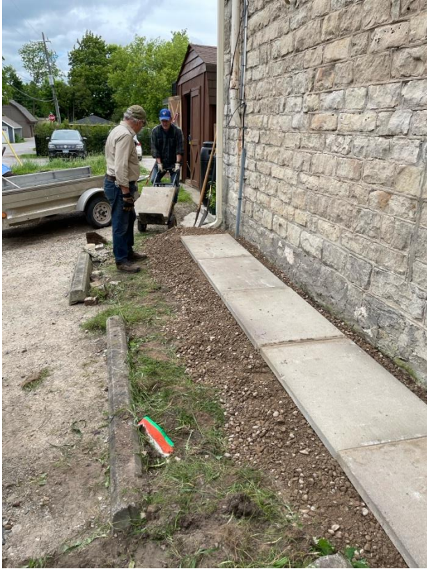
Preparation of the pad for the rain barrels
