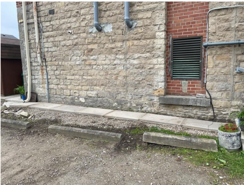
Completed base for the rain barrel series
