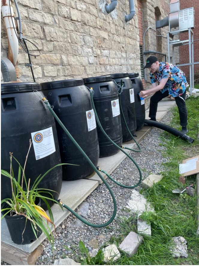
In mid August the signage was applied to each rain barrel.
