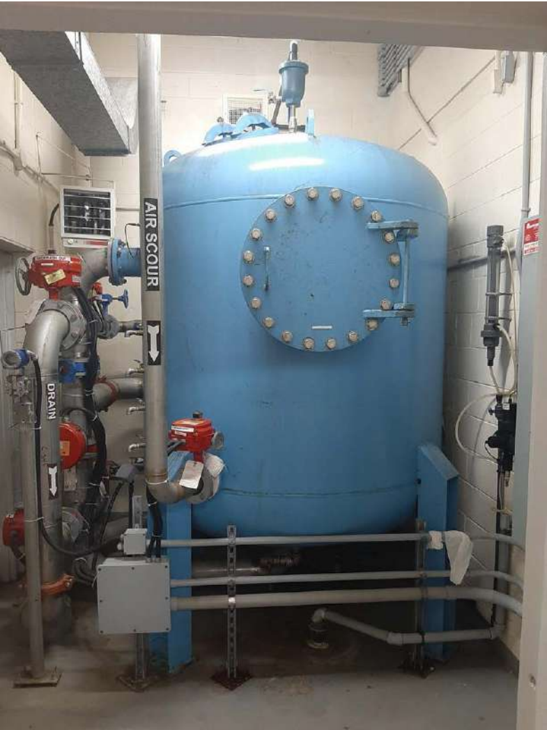
Well 8B/8C Filter Vessel
