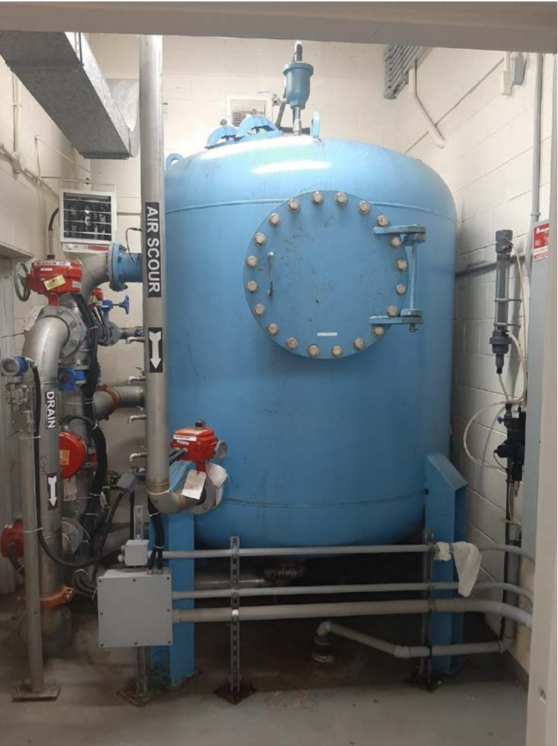
Well 8B/8C Filter Vessel
