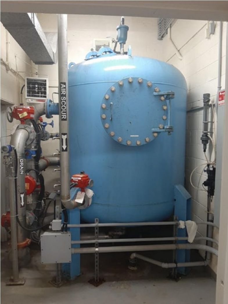
Well 8B/8C Filter Vessel
