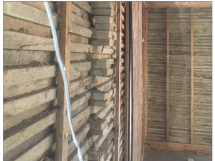
Interior view showing the offsetting of the planks to receive plaster, and remnants of former plank-on-plank partitions. (City of Markham, 2018)
