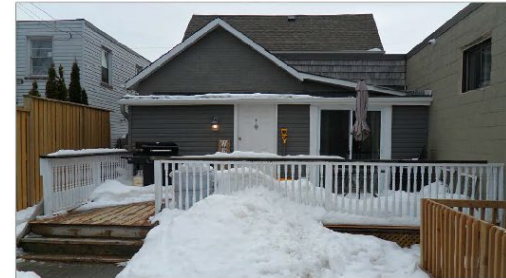
P-5 REAR EAST END LOOKING SOUTH
