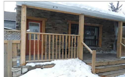
P-6 REAR WEST END LOOKING SOUTH
