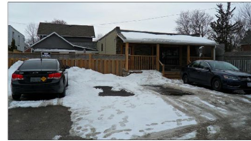
P-4 REAR LOOKING SOUTH
