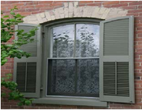
Original two-over-two sash windows
